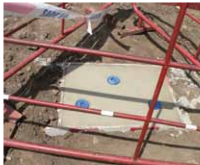
Three of the more than 500 street covers
