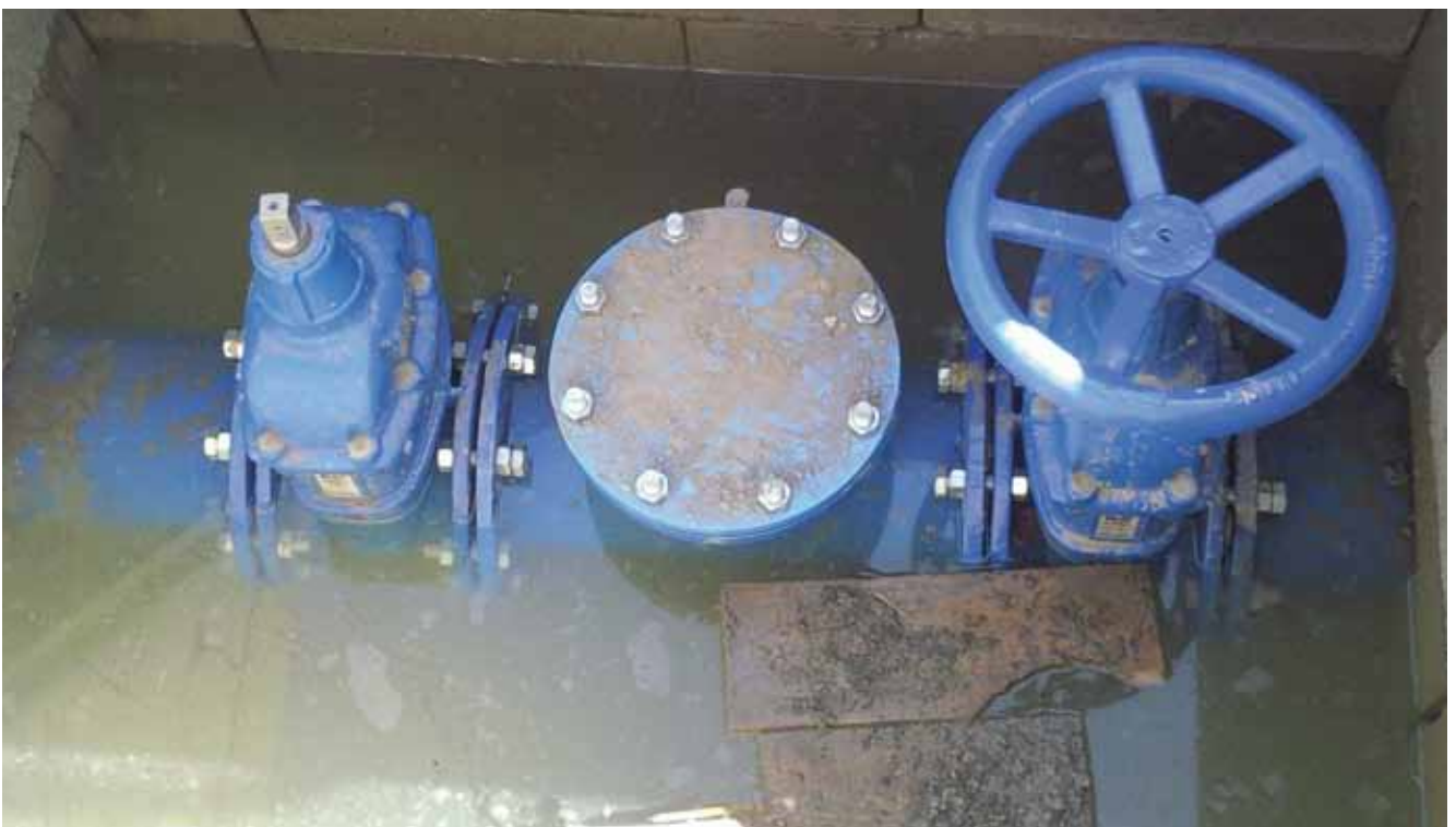
A recently installed gate valve
