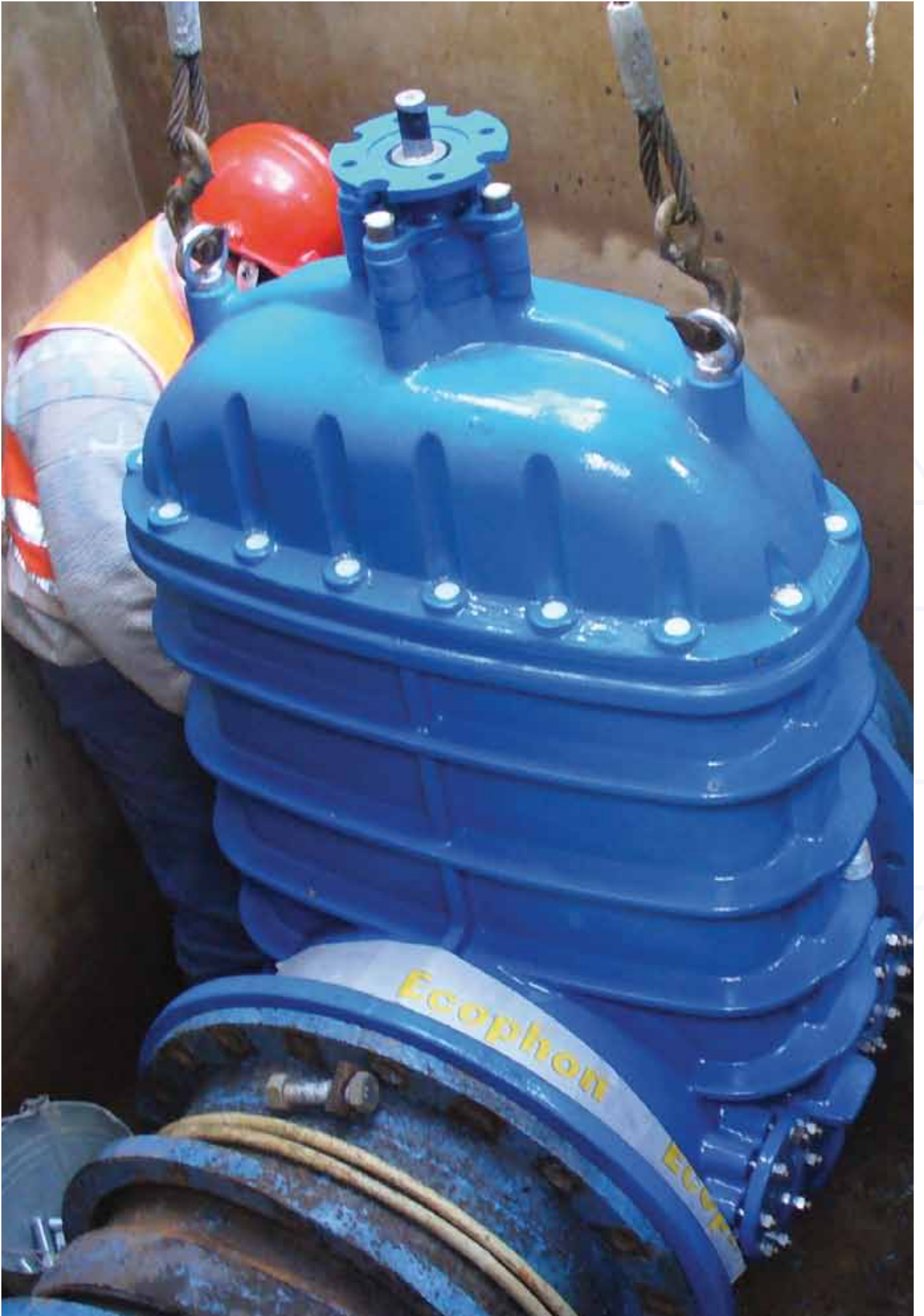
Water network reconstruction in Hungary Sent in by Kornél Oberding, Euroflow
