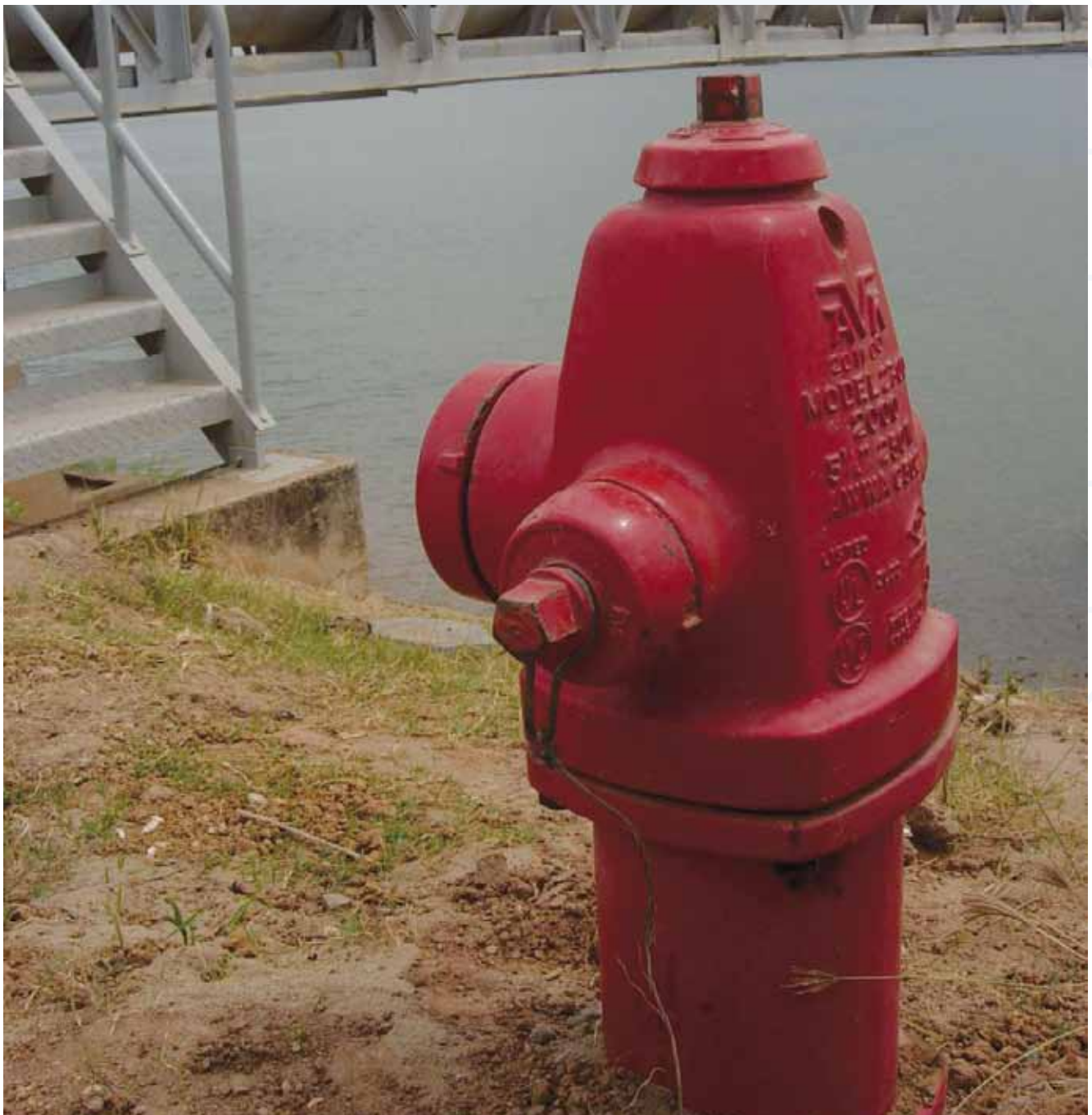
AVK series 27/00 Dry Barrel Hydrant 9 years after installation. Manufactured by American AVK and supplied by AVK Malaysia. Installed at Water Intake of Chruoy Chang War Water Treatment Plant, Cambodia.
