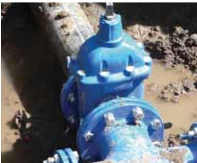
A recently installed gate valve
