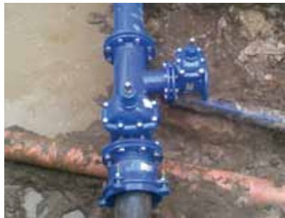
Renovation of an old pipe to new AVK valves and AVK ORION Sent in by Frantisek Sramek, sales manager AVK VOD-KA a.s.
