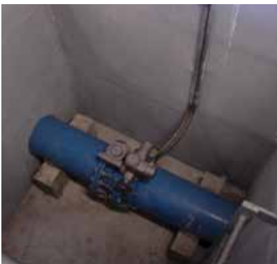
AVK concentric butterfly valve with electric actuator
