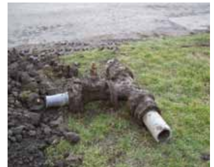
One of the valves that was replaced
