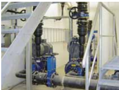
Project in Norway, Series 702 knife gate valves and Series 53 ball check valves Flemming Bindslev, Krüger A/S
