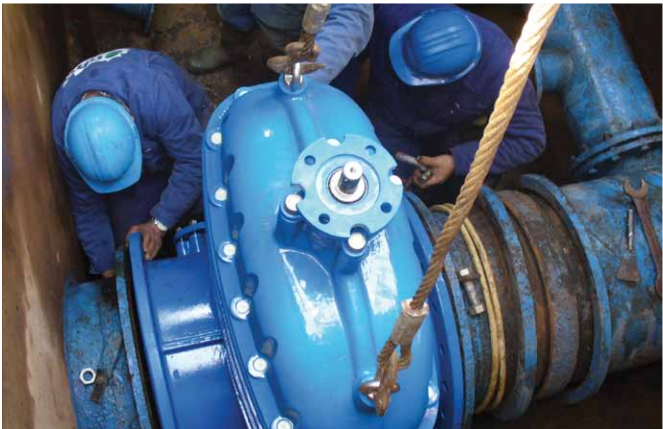
The new DN 600 gate valve is being installed
