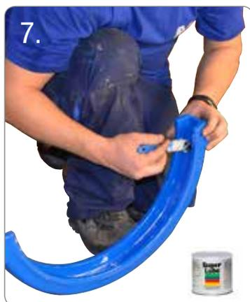
Before mounting the brackets use suitable lubricant, e.g. drinking water approved silicon grease, inside the bracket.
